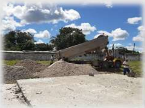
Three truckloads of sand delivered so far
