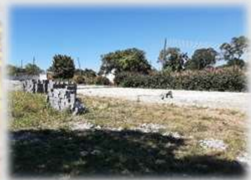
Materials on site – ready for the bricklayers to arrive
