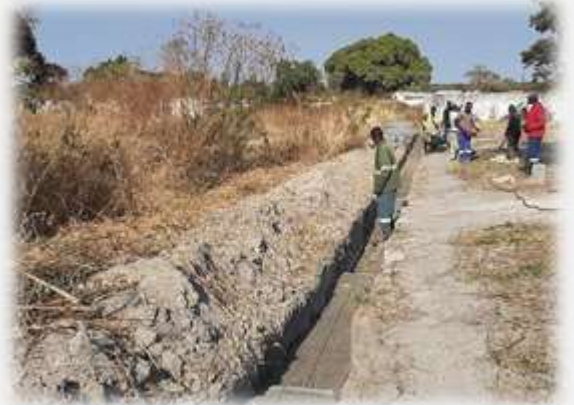
Our new perimeter wall being built in the August holiday
