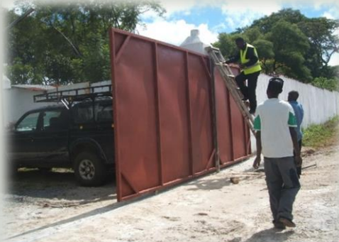
Installing the gate
