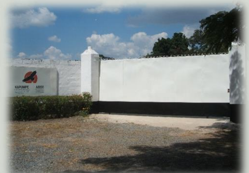
Finishing our gate with paint
