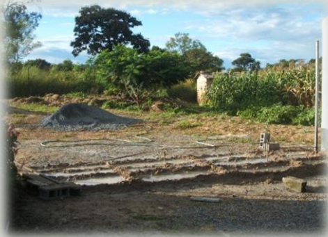
Laying foundations for the gate
